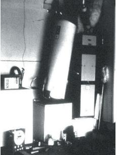
**Figure 11** - This unstrapped water heater tipped over during the 1984 Morgan Hill Earthquake. Fortunately gas and water lines were not ruptured.
