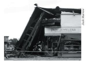
Figure 6 - San Simeon Earthquake, Dec. 22, 2003. The Acorn Clock Tower Building constructed of unreinforced masonry collapsed killing two people.
