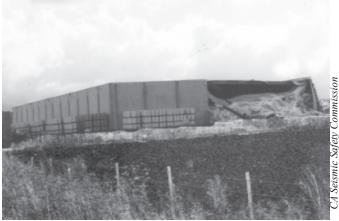
**Figure 41** - Pallets of canned goods stored in this building fell off the shelves during the 1989 Loma Prieta earthquake and pushed out the concrete wall of this Hollister warehouse.
