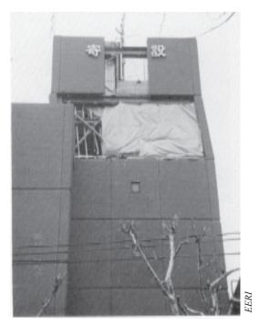
**Figure 29–**A six-story steel braced frame building was damaged after the 1995 Kobe Earthquake in Japan. 4,000 to 8,000 small commercial buildings and 1,000 to 2,000 large commercial buildings were destroyed or severely damaged in that event.
