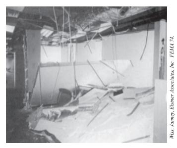
**Figure 60 -** Partitions and ceilings toppled onto office spaces during the 1994 Northridge Earthquake.
