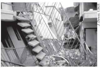
**Figure 36** - Stairs to an apartment building collapsed during the 1994 Northridge earthquake.
