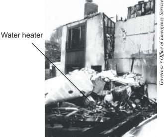
**Figure 10** - The unbraced water heater in this building fell during an earthquake; the resulting fire destroyed the building.
