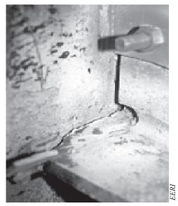
**Figure 27–**This steel frame connection unexpectedly cracked in the 1994 Northridge earthquake.
