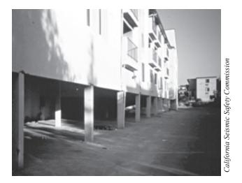
**Figure 30–**Apartments with tuck-under parking like this can collapse. This building is leaning but did not collapse in the 1994 Northridge earthquake.
