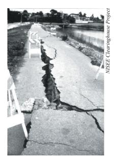
**Figure 67 - Lateral Spreading.** Loma Prieta Earthquake, October 17, 1989. Lateral spreading damage levee road along the San Lorenzo River.
