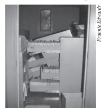
**Figure 3** - File cabinet drawers can slide open and unbolted cabinets can topple during earthquakes.
