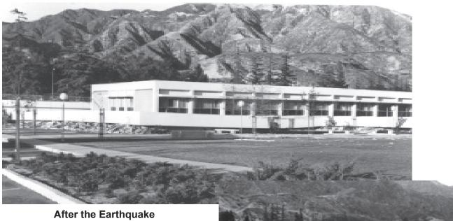
**Figure 25 -** The walls and columns holding up the Psychiatric Unit of the Olive View Hospital weren't adequately reinforced; they collapsed in the San Fernando Earthquake of 1971. It was a two-story building before the earthquake. Only because the earthquake occurred during an early hour of the morning, the building was fortunately not occupied and a large loss of life was avoided. This type of construction is common in older California commercial and institutional buildings.
