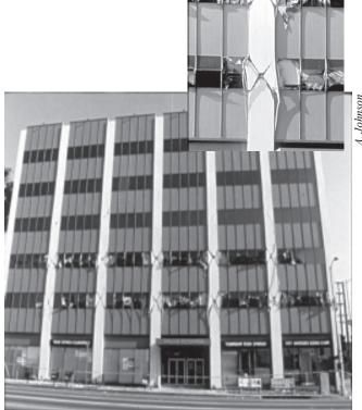
**Figure 23 -** This medical office building's exterior cladding affected the way its frame responded to shaking, and the columns failed during the 1994 Northridge earthquake. The building was demolished and all medical records inside were destroyed.
