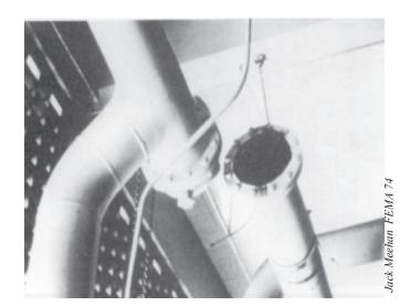
**Figure 47** - This pipe joint separated during the 1971 San Fernando Earthquake.
