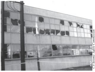
**Figure 56–**The windows in this San Francisco building probably broke because its frame flexed too much in the Loma Prieta earthquake of 1989.
