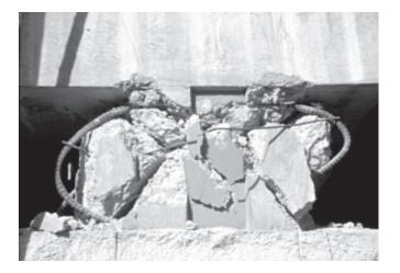
**Figure 22** - Short columns in this parking structure failed in the 1994 Northridge earthquake. Modern building codes now require much more reinforcing steel for such short columns.
