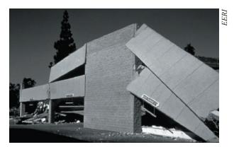
Figure 5 - Concrete Parking Structure Collapse.
