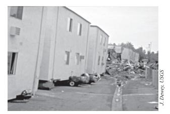
**Figure 31–**A similar apartment building's soft story collapsed on cars during the same earthquake.
